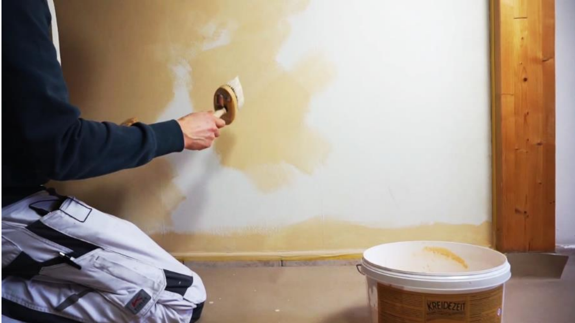
An example of the application of paint in cloudy, irregular masses of varying sizes, and on diagonals.
