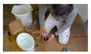
• Once the mixture is homogeneous, mix it with the lime plaster previously mixed with water (as described in step 3).
