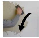
• Apply the plaster starting from the top of the wall, in sections of about 10 to 15 sq.ft., to the bottom of the wall. Repeat the operation over the entire wall section, while ensuring to work *al fresco* (don't leave it to dry during the application to ensure smooth transitions).
