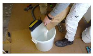
• Stir with an electric drill fitted with a powerful mixing attachment until blended. Leave to stand for at least 15 minutes, then stir again before use.
