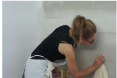
• Starting from the bottom and working your way up the wall, apply the casein primer evenly – and in cross movements – saturating the substrate. Apply only the amount of liquid that can be absorbed by the surface. Remove excess (wet shiny spots) with a cloth <u>before</u> drying.
