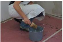
If the surface is composed of different materials (drywall, plaster joints, for example), first treat the plaster joints, ensuring they are saturated. Let them dry for 8 hours before applying the casein primer to the entire surface. Remove excess (wet shiny spots) with a cloth <u>before</u> drying.
