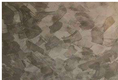
Thanks to the overlapping, the typical structure of a spatula application is created. Colors appear more evenly after drying.
