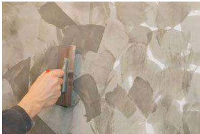
Application of the second layer.
