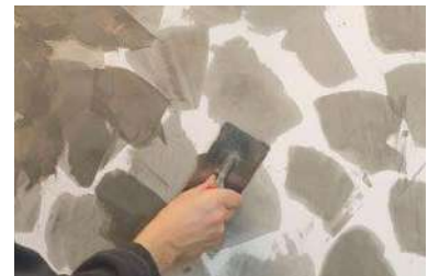
After applying the initial patches, additional patches are applied in between.
