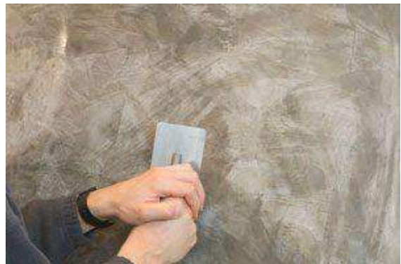
The soaped surface is troweled under pressure.
