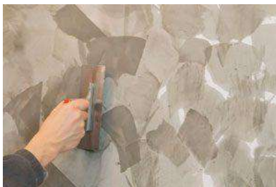
Third step, the remaining gaps are covered.
