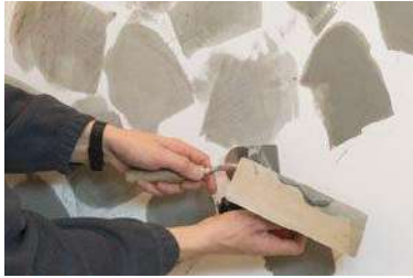
Work with only a small amount of material on the trowel.
