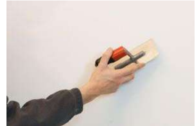
The slight imperfections in the 0.5 mm lime wall finish are scraped off using the trowel.
